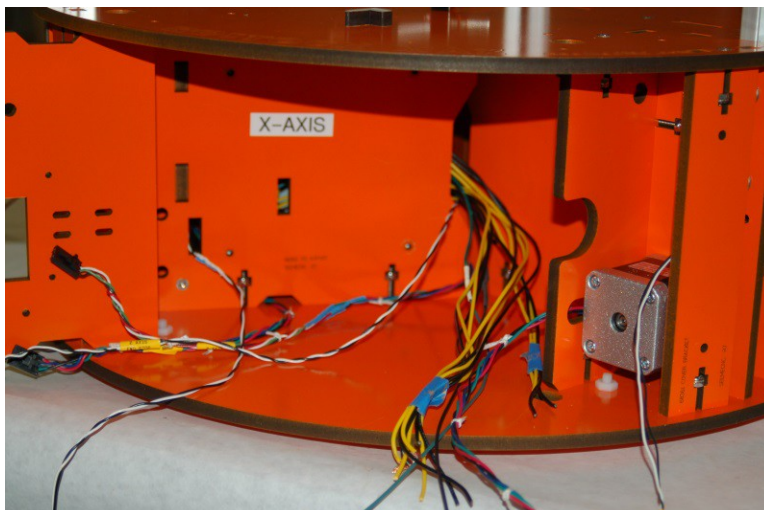
Fig. 13-4: Power wires routed to the electronics bay.
